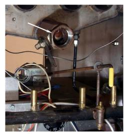
Ball retainer nut (arrow) on drain valve.
